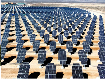
Solar power generation(DC to AC)
