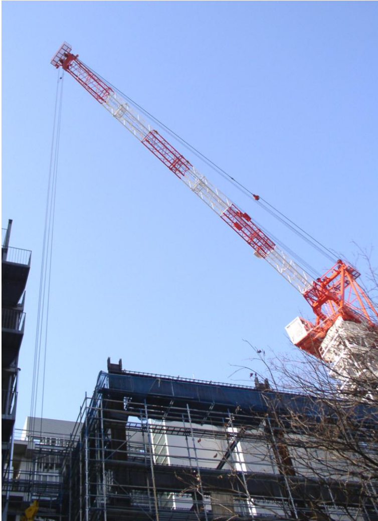
1-3; a Climbing Crane ( Torque )
