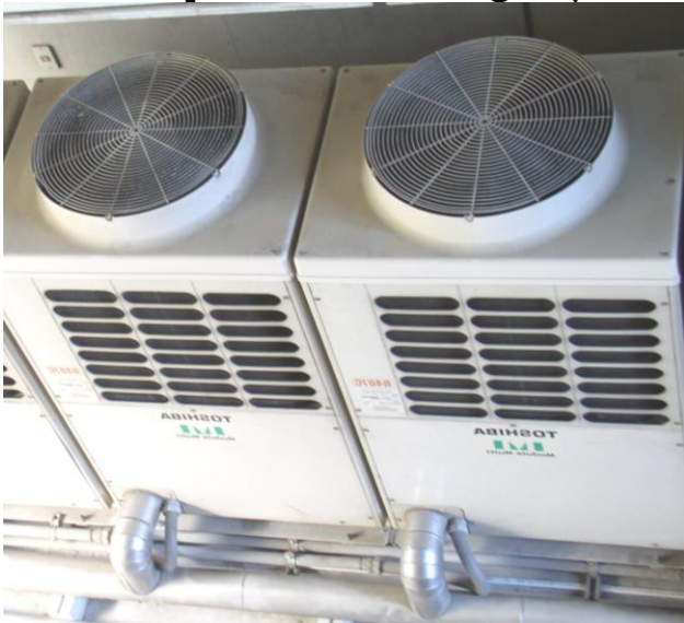
11-3(a); a Heat exchanger of a Heat Pump. @ Nagoya University.
