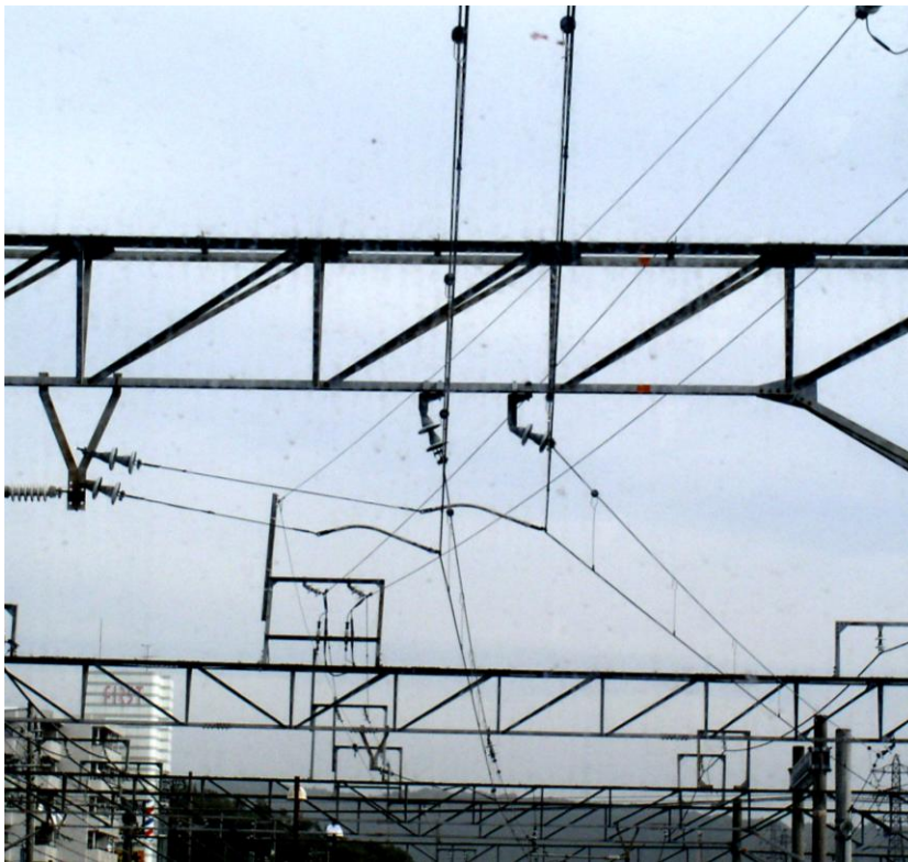
1-1; 電車の架線の切り替え(a relay of the electric string cables, @ JR-Kozoji Station.
